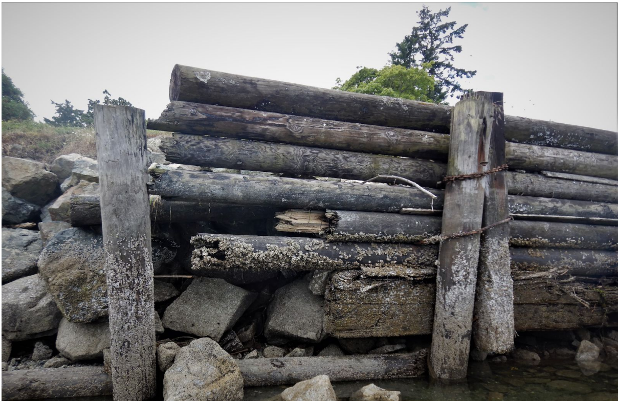
Example of a creosote-treated log polluting feature and a sea wall in poor condition.
