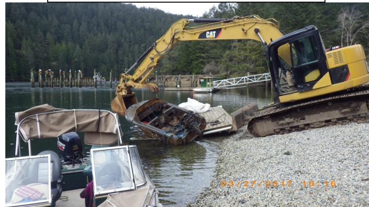
Excavator removing one of the derelict vessels from the work float to load into a debris bin
