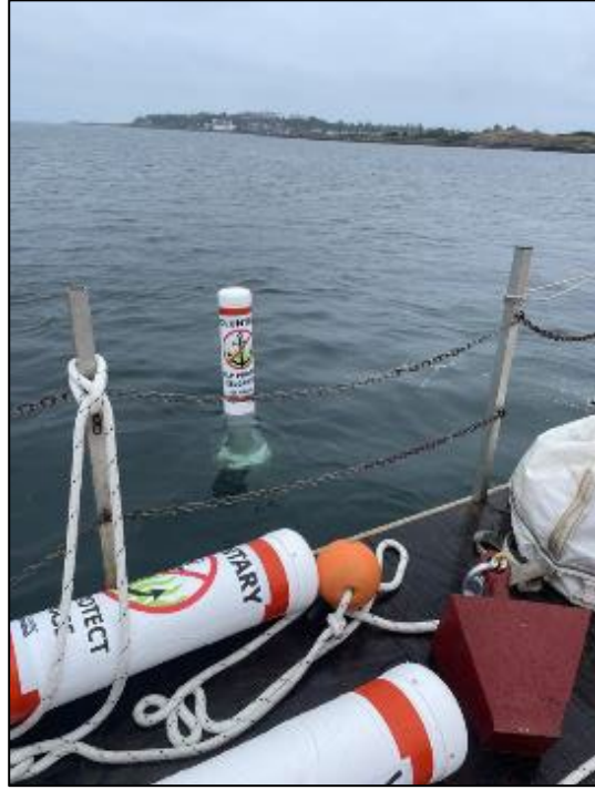
Figure 19. Deployment of the “Voluntary No Anchor Zone” buoys. A crane on board the Collective Effort drops the anchor block into the sea. The buoy is attached to the mooring block with a mid-line buoy system, which keeps the line from scouring the seafloor. Photos by J. Smith.
