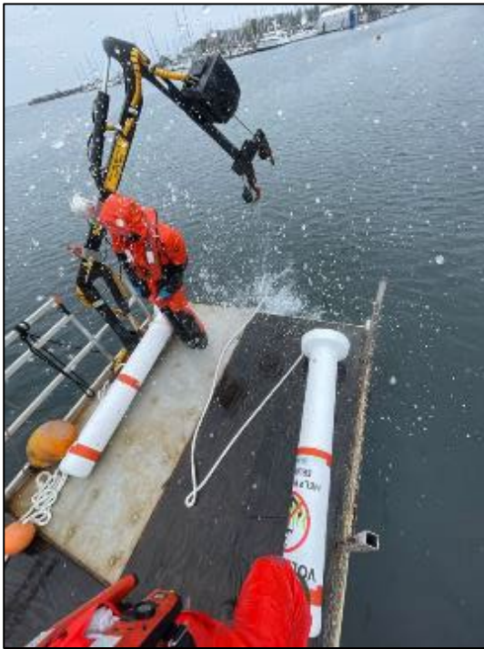
Figure 19. Deployment of the “Voluntary No Anchor Zone” buoys. A crane on board the Collective Effort drops the anchor block into the sea. The buoy is attached to the mooring block with a mid-line buoy system, which keeps the line from scouring the seafloor. Photos by J. Smith.
